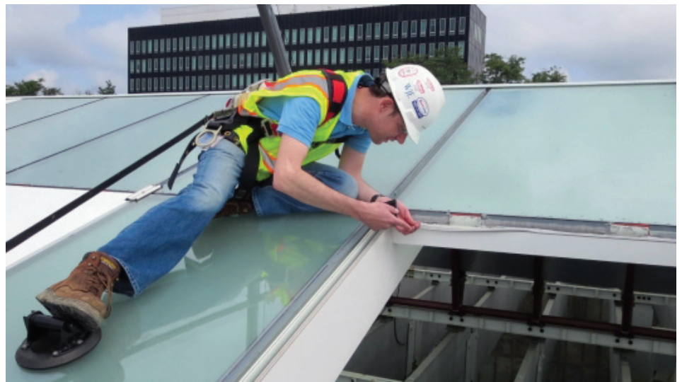
FIGURE 1 A fully integrated BECx process can result in overall, long-term cost savings.
